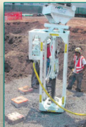
A-2 Vertical Equipment mounted drill used for drilling on foundations.
